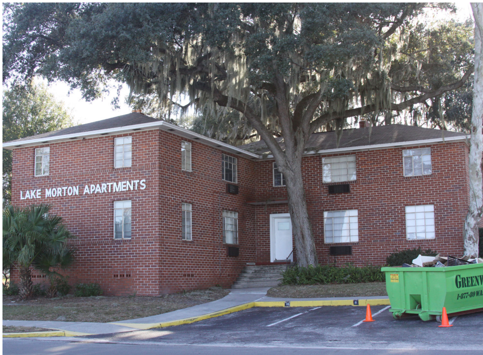
Renovations began on the future FSC housing on Lake Morton.
